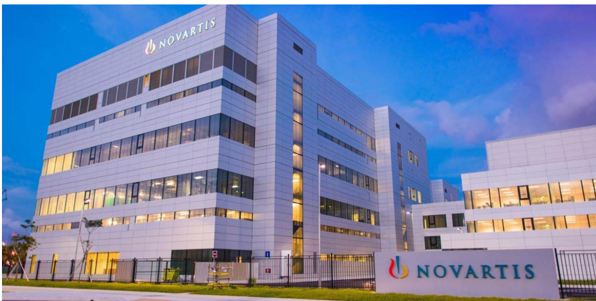
Novartis Singapore manufacturing plant.
